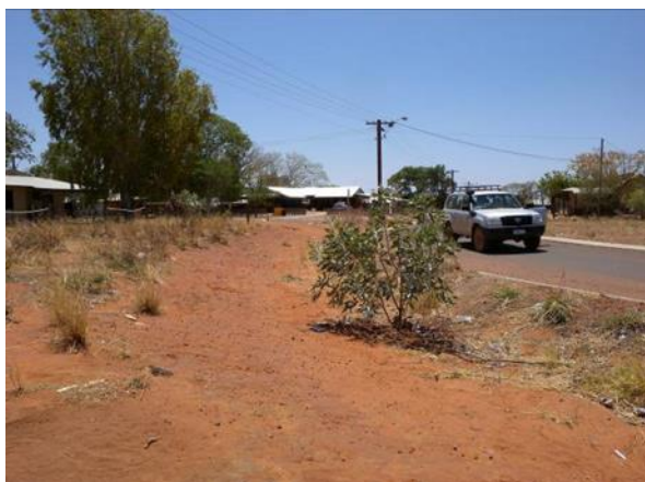
Figure 7 - Yaruman Road Drainage Channel
