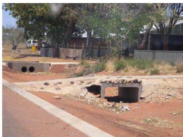
Figure 8 - Constructed Culverts over drainage channels
