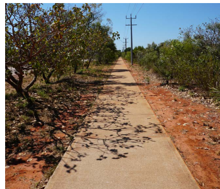
Pedestrian and cycling footpath along Cable Beach Road West
