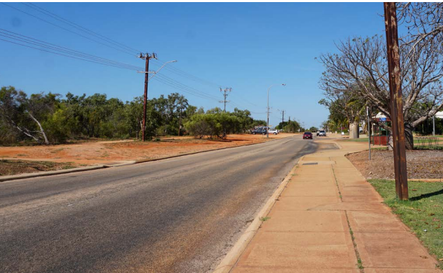
Sanctuary Road Concept - Existing Conditions
